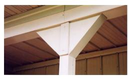
The header is trimmed using 1 piece of trim that covers the front, bottom and back of the header.
