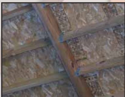
OPTION: Purlins in clips eliminate bird nesting.
